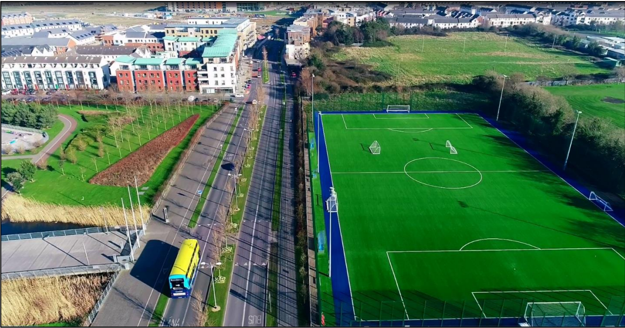
Fig. 3 – Drone Photo depicting existing infrastructure in place at Clongriffin including Father Collins Park
