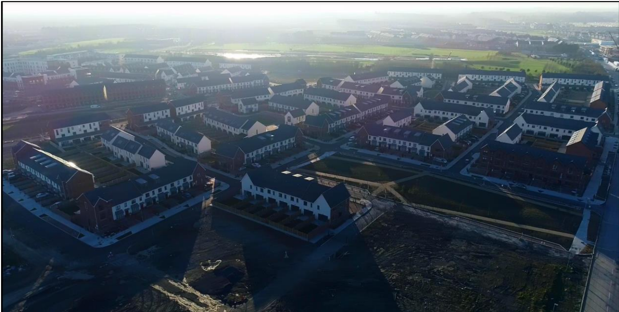
Fig. 5 – Drone Photo depicting existing residential units constructed and under construction at Clongriffin
