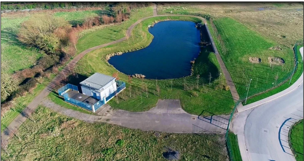
Fig. 4 – Drone Photo depicting existing infrastructure in place at Clongriffin including aspects of the River Main Corridor
